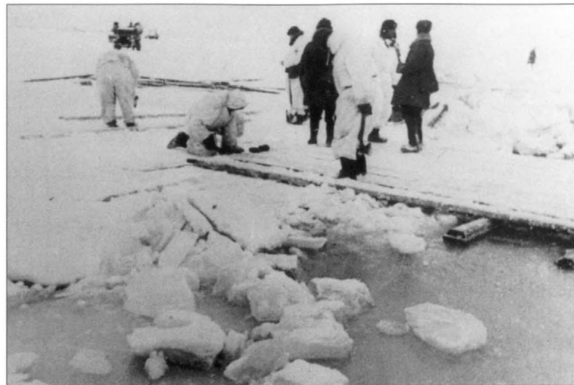
ABOVE: Although communications with the outside world had been established by the end of 1943, the "Road of Life" was not immediately redundant. With their transport parked carefully on thicker ice, this section of Red Army engineers gingerly inspects a weak point. Groups such as this worked around the clock and in all conditions to maintain ice routes.
