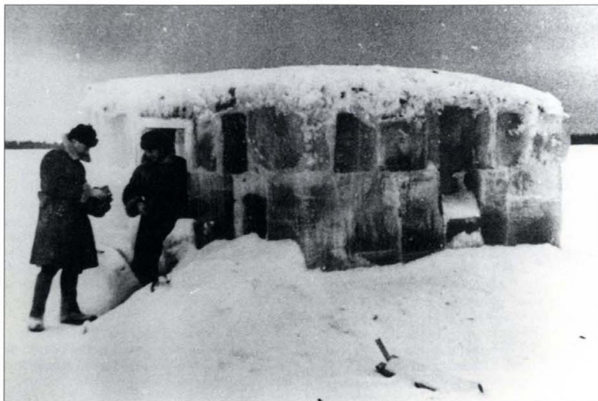
ABOVE: An essential feature of the “Road of Life” was the thickness of the ice. The Red Army’s meteorological branch performed a vital, if ungung , service from isolated stations such as this ice-block hut dotted across Lake Ladoga.
