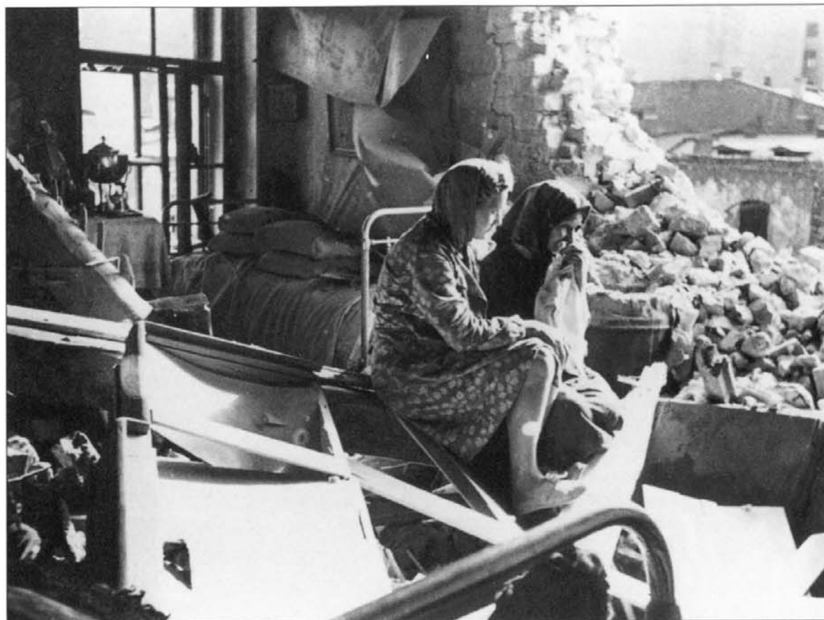
ABOVE: On 20 August 1942, tragedy struck the Amelkin family – their apartment was heavily damaged by enemy fire. The thickness of the wall must have absorbed much of the explosion as the furniture and the family samovar are almost undisturbed.
