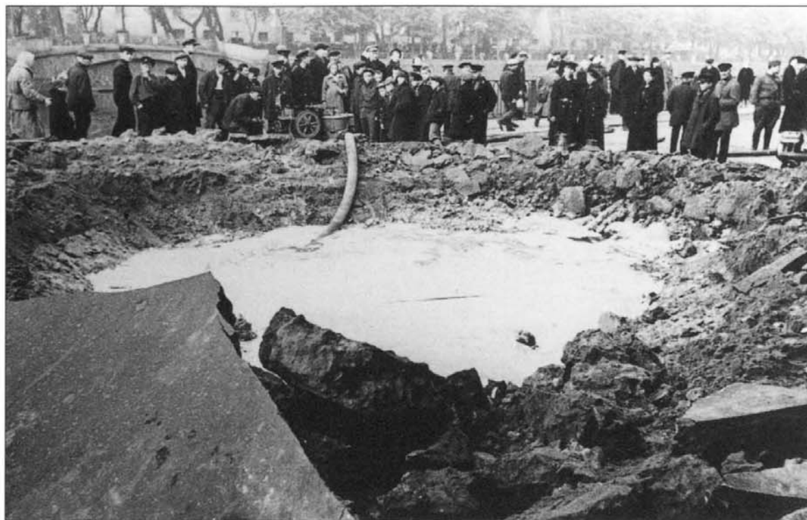
ABOVE: This photograph was taken in September 1941, when the novelty of bombing or shelling was such that it would attract a crowd of onlookers. The pump is emptying the crater so that the water mains can be repaired.
